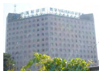
Figure 1. Central building of the Chinese Academy of Sciences (CAS) in Beijing.
