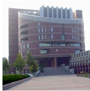
Figure 3. Main building of the Institute of Physics, Beijing, CAS.
